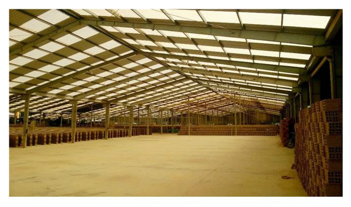
All primary and secondary structural components are cut, punched, drilled, welded and formed into the front in the factory before being transported to the site. The quality of home components is always guaranteed because it is fully manufactured at the factory according to standards and strictly tested. At the construction site, prefabricated components at the factory will be linked together by bolts.
